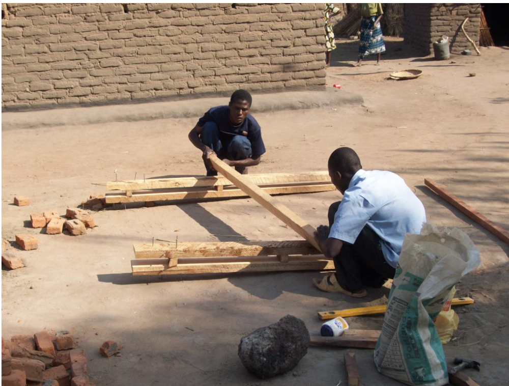
Figure 3.12: Alinafe and Happy Constructing the Abakus Pole System
